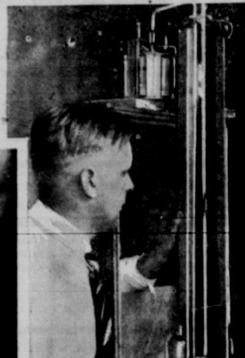
MEASURES NOTHING: Impossible? Not so modern science. This device checks the vacuum in cans of coffee packed by the newly discovered vita-fresh process, to make sure that oxygen, enemy of coffee flavor, does not exceed two tenths of one per cent.
