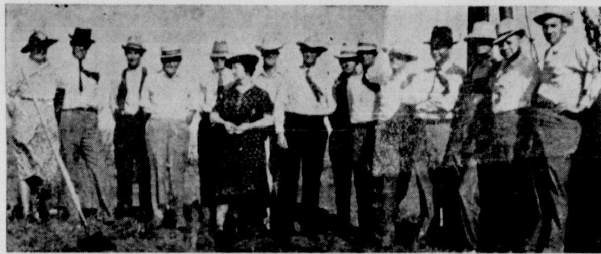
PIONEERING IN RURAL ELECTRIFICATION —Above are members of the board of directors and officials of the Hall County Electric Co-operative, pictured as they watched the first poles set on the 113-mile REA line which will be opened Saturday. Left to right, they are: Mrs. C. A. Williams, Paul Montgomery, Clyde Fowler, Tom Lenoir (secretary of the board), Harry Tyler, Mrs. N. A. Hightower, Harold Hodges, Jake Lamb (vice president), I. V. Sharlach (construction superintendent), Edgar Foster, B. L. Gresham, R. D. Hall (president), C. M. Hawkins, Otho Fitzjarrald (attorney), and Alvis Yarbrough (project superintendent).
