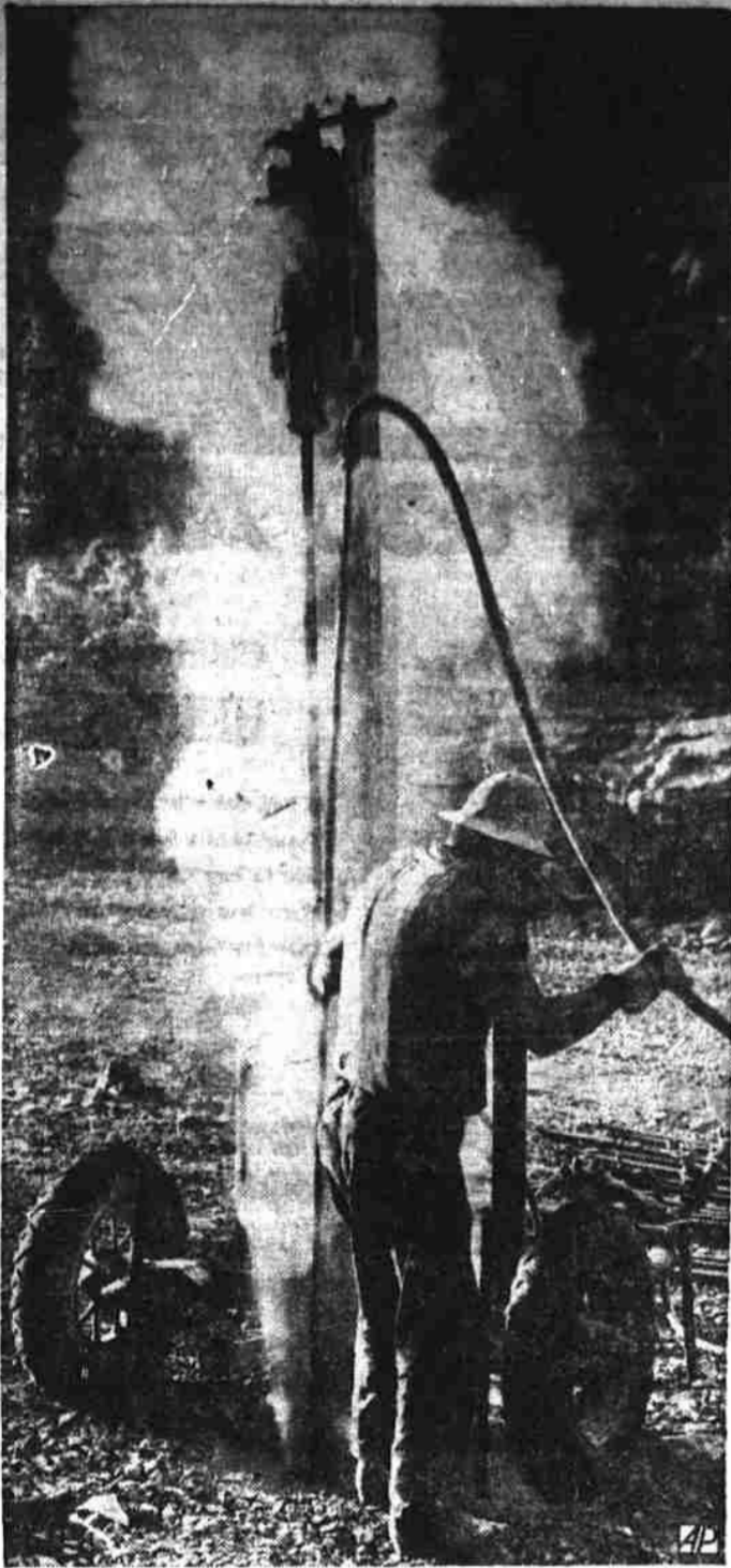
MAN-MADE GEYSER spouts rock dust at the site of a temporary diversion channel—part of the Shasta dam project on the Sacramento river, California. The workman has turned a stream of air into the hole to clear it of rock dust. The hole he is drilling is to be used to blast out rock in the canyon, where the dam is being built by the U. S. bureau of reclamation.
