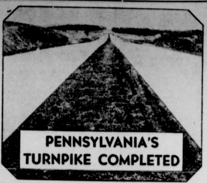
For 160 miles the Pennsylvania Turnpike stretches on like this, with few curves and no grade intersections.
