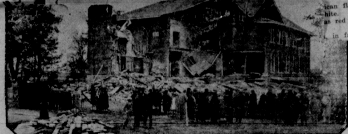
The dynamite-torn schoolhouse at Bath, Mich., where 36 pupils and five adults were killed when the building was dynamited by Andrew Kehoe...
