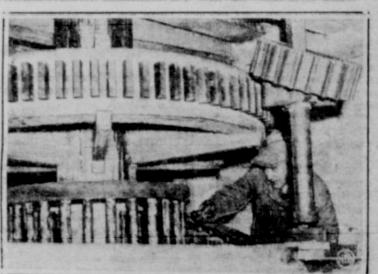
At a cost of \$19,200, the old Isaac Pierce mill, in Rock Creek Park Washington, D. C., is being restored to working condition by the WPA oft was built in 1819, but 60 years later was abandoned because the machinery was worn out. A mechanic is pictured below putting the restoring touches on the wooden gears that are driven by the huge waterwheels. In recent years the mill (top) has been a tearoom
