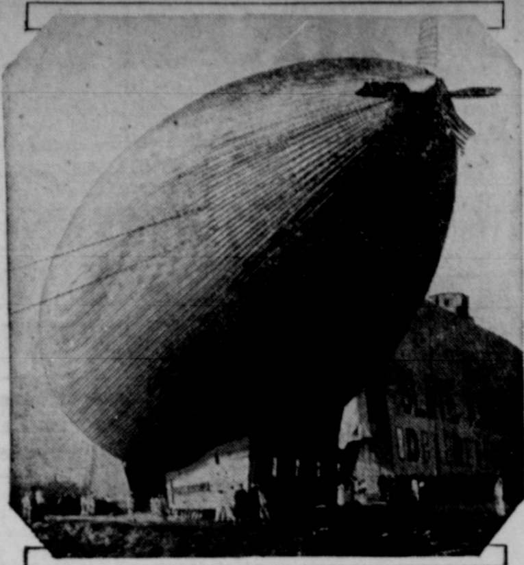
Here is the City of Glendale, the world's first all-metal steam driven dirigible, as it appeared when first drawn from its hangar, at Glendale, Calif. As soon as the work of installing motors is finished, the strange craft will undergo a test flight. It is made of duraluminum, the strongest metal for its weight known. Captain T. B. Slate, builder and designer, says it is the first of a fleet of trans-continental air liners.
