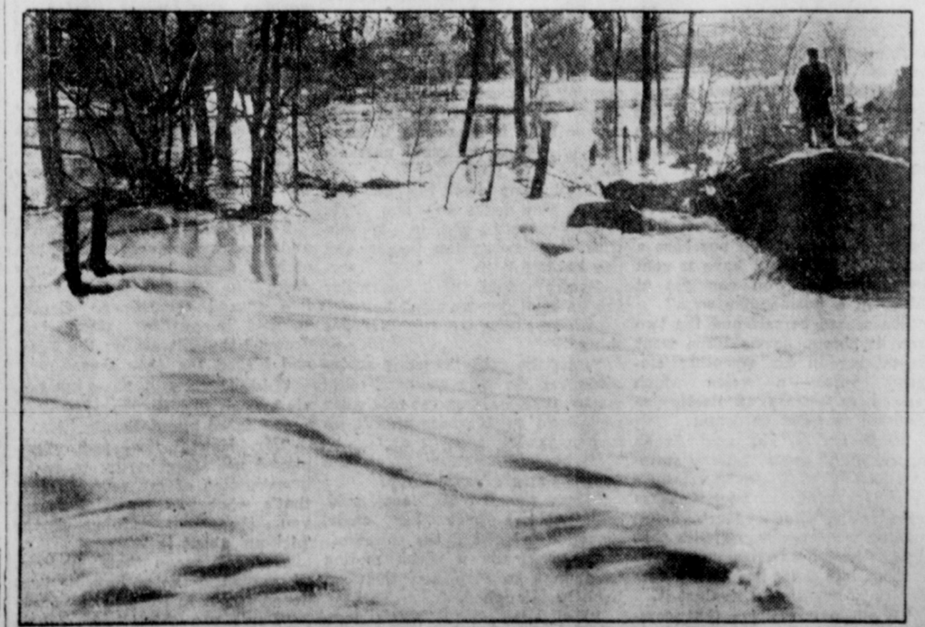
A dynamite explosion which ripped open this levee near Philipp, Miss., freeing torrents of the Tallahatchie river, brought militiamen rushing to the scene, to halt further blasting by upriver planters, whose lands had been flooded by high waters. Heavy property toll was taken when the river went far out of its banks, in the series of floods which have ravaged eight states.
