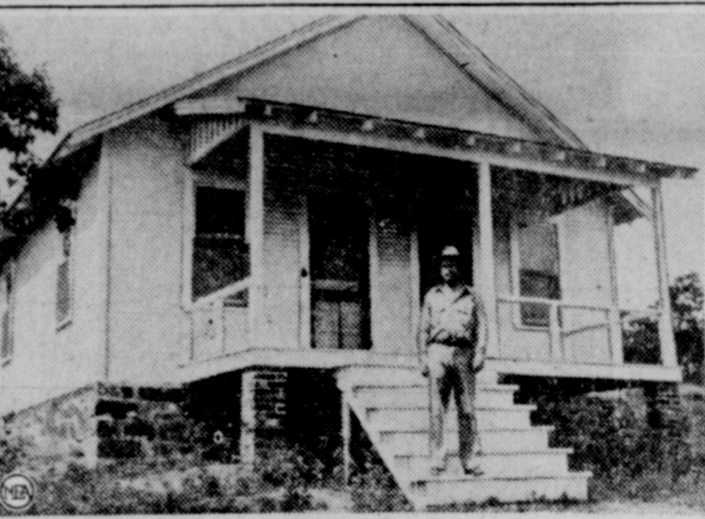
A federal relief project for Indians will "rescue" the John Battiest family from the shack in front of which they are pictured in the top photo and move them to a clean, comfortable dwelling of the type shown below. They will be among the Choctaws and Chickasaws to benefit by the colonization plan at McCurtain, Okla., nearly completed, in which homes and farming tracts will be provided for indigent Indians. On the steps of the home in the bottom photo is Henry Nicholson, project building chief.
