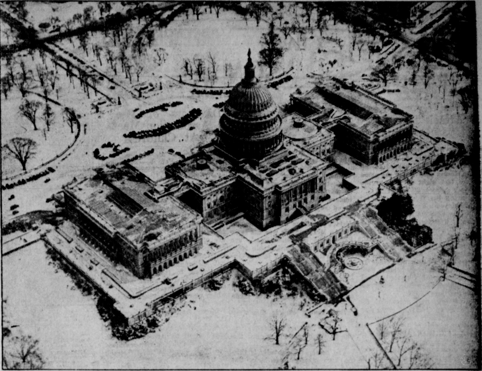
The blizzard sweeping across much of the country left the Capitol grounds in Washington under an unusual 11-inch blanket of snow, and gave a flying photographer a chance to make this unusual picture of the Capitol and its surrounding grounds. Note the rows of autos parked in the oval Plaza before the Capitol building, and how clearly this aerial top-side view marks the division of the two wings, Senate on the left, House on the right, of the ancient building.
