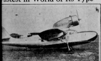
ands out in every line of this huge trim ship, the largest single-engined amphibian transport in the world, the er, just completed for the Pan American Airways Sysarrying two pilots, eight passengers, and 1000 pounds of he craft can attain a cruising speed of 158 miles an hour. art of the craft is streamlined, the main wheels retractwith the underside of the wing to eliminate resistance ven the wing tip floats and the tail wheel retracting.
