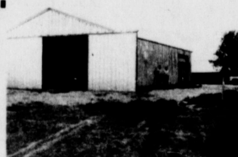
Bob Smith and Bill Schuette beside the building constructed on the Schuette farm east of Canyon.
