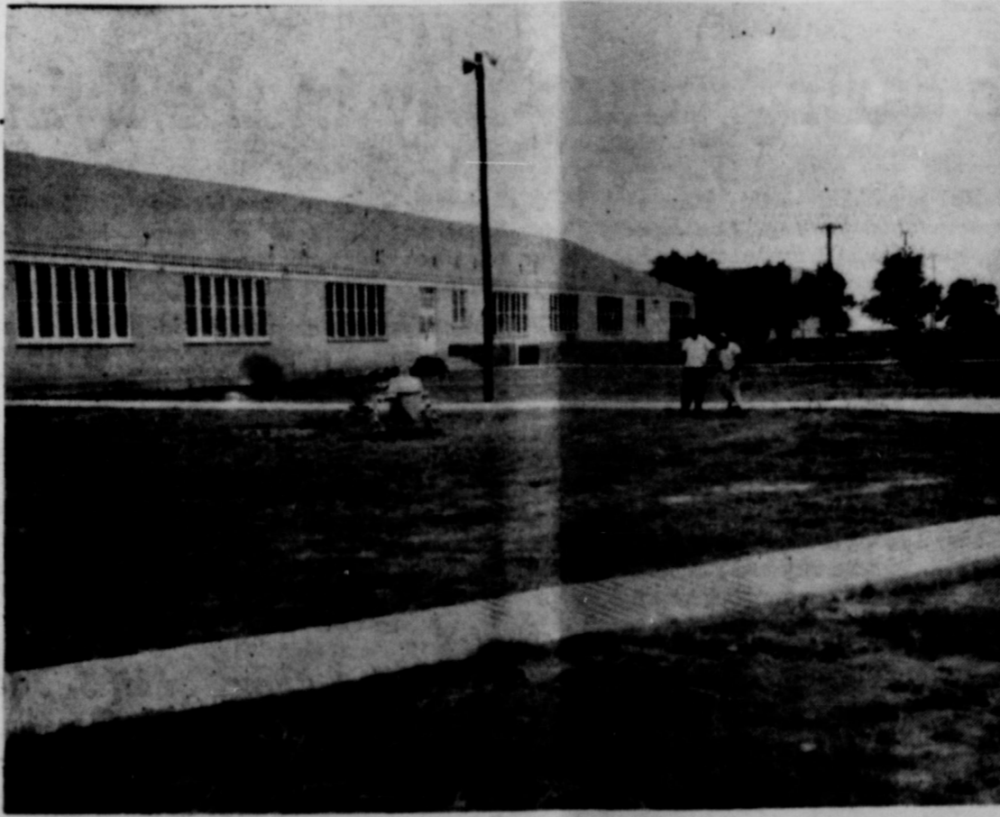
LOOKING OVER THE BACK YARDS — At the Springlake High School is Supt. Bill M... and Ed Haley. Much of the yard improvements, and construction of wall and other projects have been donated by Earth and Springlake civic clubs.
