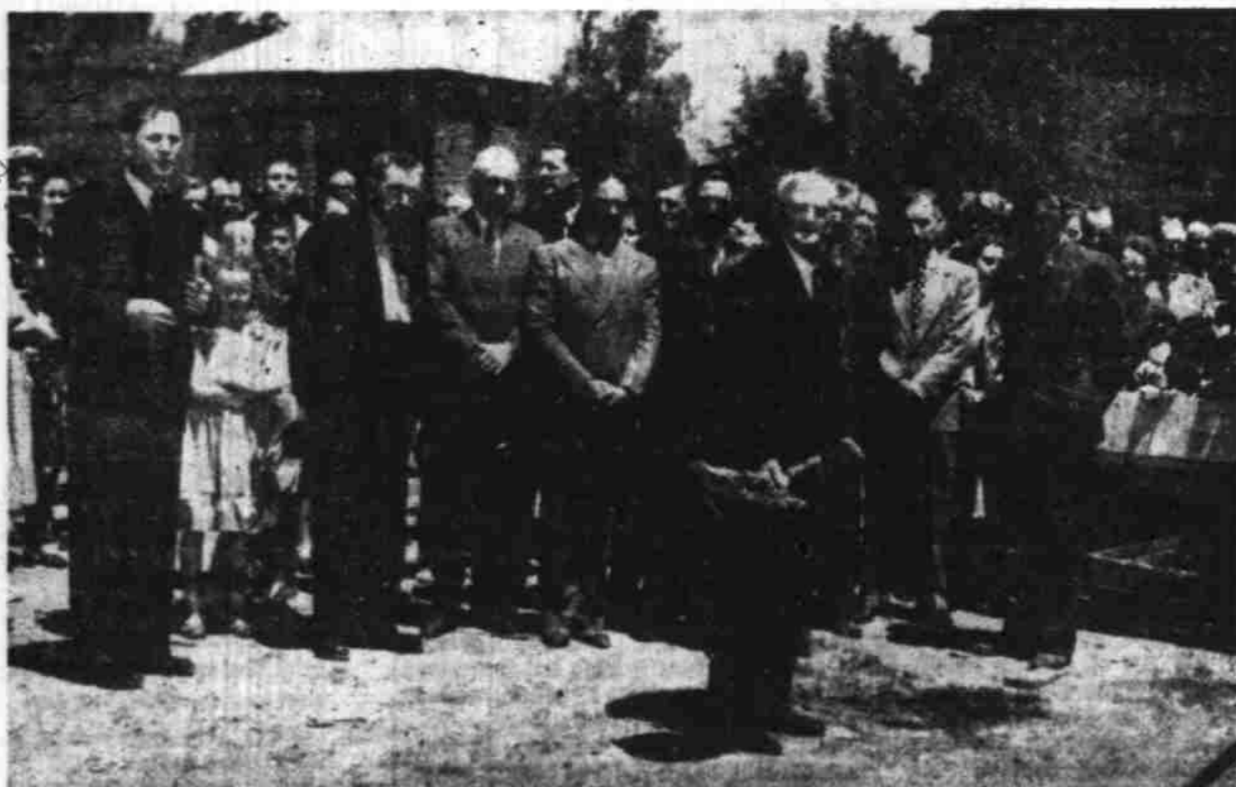
A TEMPLE BEGINS.—J. R. (Jim) Sales, senior deacon of the First Baptist church in Stanton, digs the first spade of dirt in a groundbreaking service marking the start on construction of a new $60,000 plant for the church. The service was held a week ago following the morning worship. The new building, a frame and brick-veneer type, will provide for 25 Sunday departmentalized Sunday school rooms and other auxiliary offices, plus a spacious auditorium with balcony. Shown left to right are the Rev. Truett R. Hawkins, pastor, L. H. White, Guy Eiland, Clyde White, Emmett Pittman, L. D. Watson, Albert Louder, Grady Cross (partially obscured by Mr. Sale), Clark Hamilton and B. F. White, chairman of the building committee. Mrs. J. O. Hardin, president of the W.M.S., is between Hamilton and White. Clyde White is BTU director and Pittman is Sunday school superintendent. Not present for the picture are Ben Carpenter, John Pinkston, and J. C. Scott, board of building-committee members. (Jack M. Haynes Photo.)
