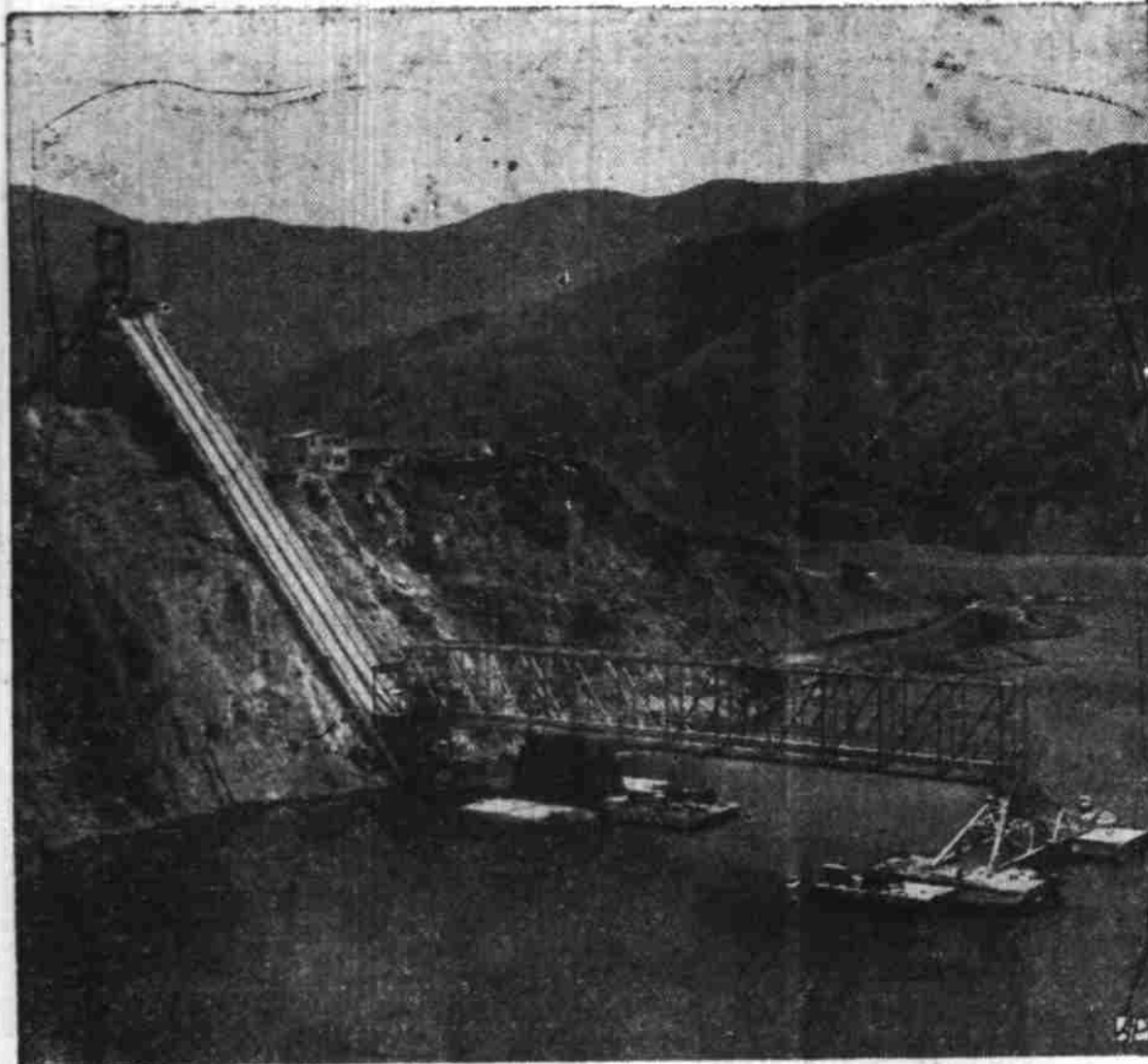
TORPEDO LAUNCHER —The Navy uses this newly-built variable angle launcher to fire test torpedoes on a man-made lake behind Morris Dam near Pasadena, Calif.
