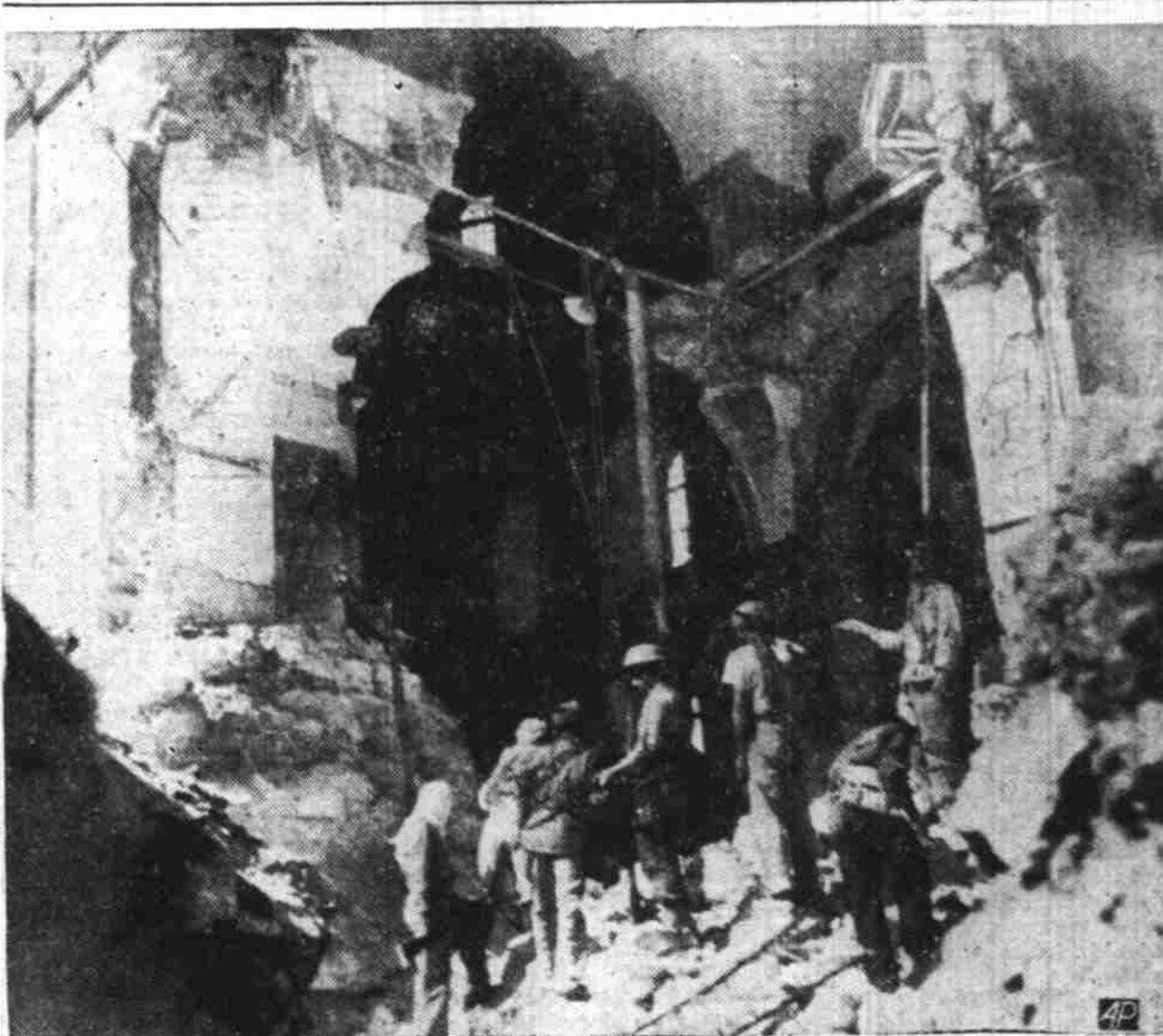
ARABS ENTER HAGANAH FORTRESS—Arab fighters pick their way through the rubble of Tiferet Synagogue, tallest in the Jewish quarter of the Old City of Jerusalem, May 21, after Arab demolition squads had blasted holes in the building which was being used as a fortress by Haganah forces. (AP Wirephoto).
