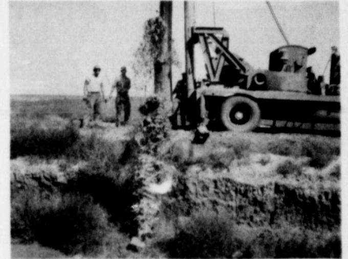
DEVELOPING A NEW HOLE WITH A 30 FOOT, 14 INCH BALER
