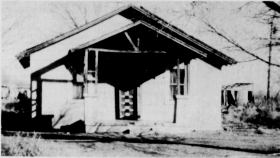
WHEN W. E. HALSELL established the town of Earth he furnished a small house to be used for school and community gatherings. It became the first church. The old building is still standing at its original site southeast of the post office.
