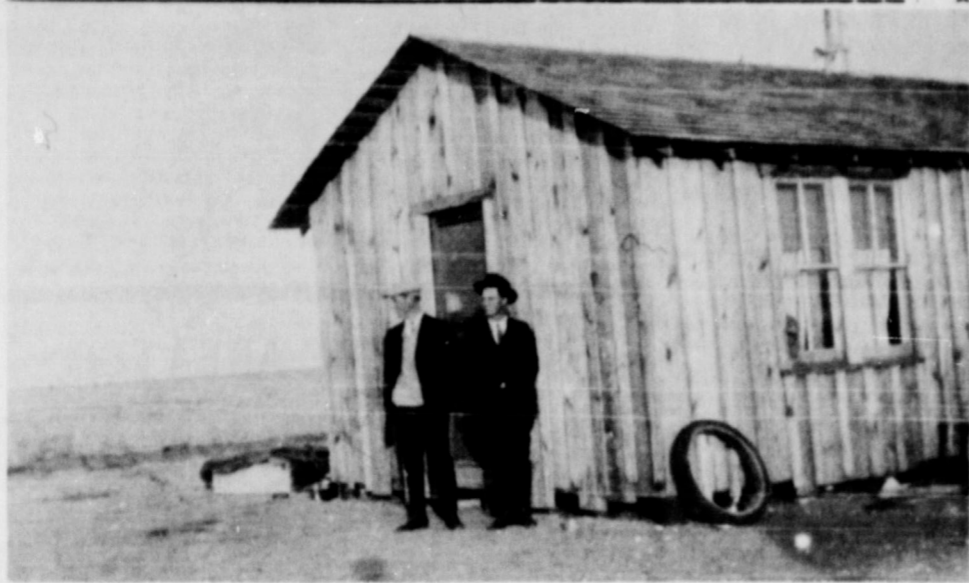
HOME SWEET HOME. The first house in Earth was purchased by Mr. and Mrs. Sam Cearley shortly after Mr. Cupp built the home. The new home consisted of one large room, without ceilings and inside walls finished. The pioneer family were so proud of their new resident.
