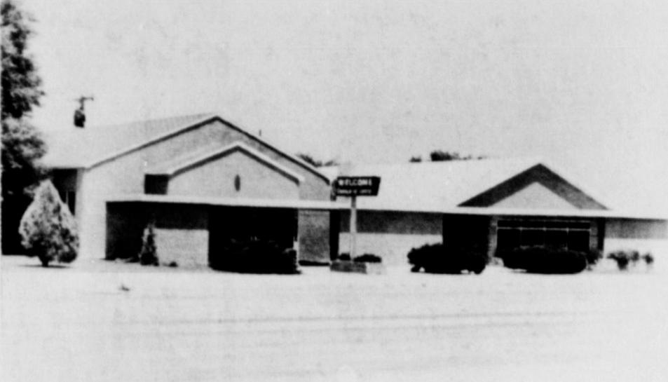
SINCE THE CHURCH OF CHRIST was first organized in 1950 many improvements have been made. The structure now has a seating capacity of 405 in the new auditorium which was added in 1962.
