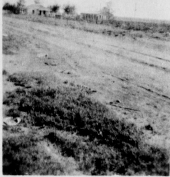
THE TWO RUT DIRT ROAD-Pictured above is Highway 70 back in 1929. The site is Earth, where the downtown section is located today. Only a few families resided here at that time. In the background is the Runyon home.
