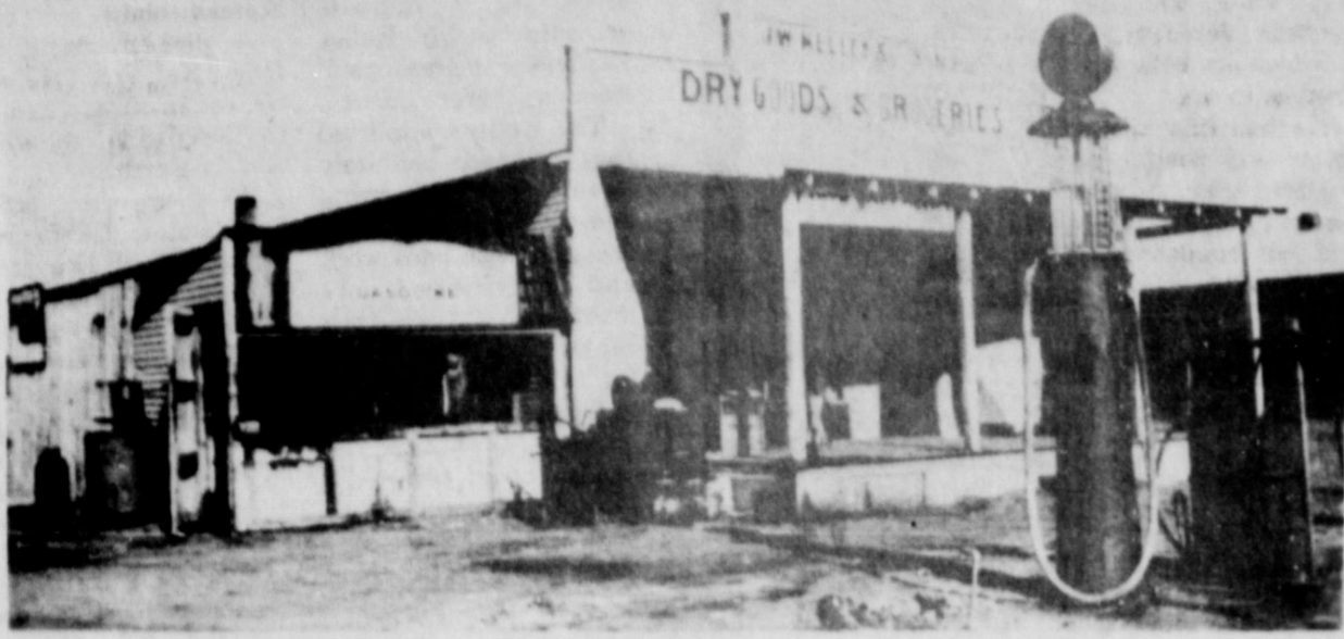
J.W. KELLEY'S & Sons Dry Good and Groceries in 1926
