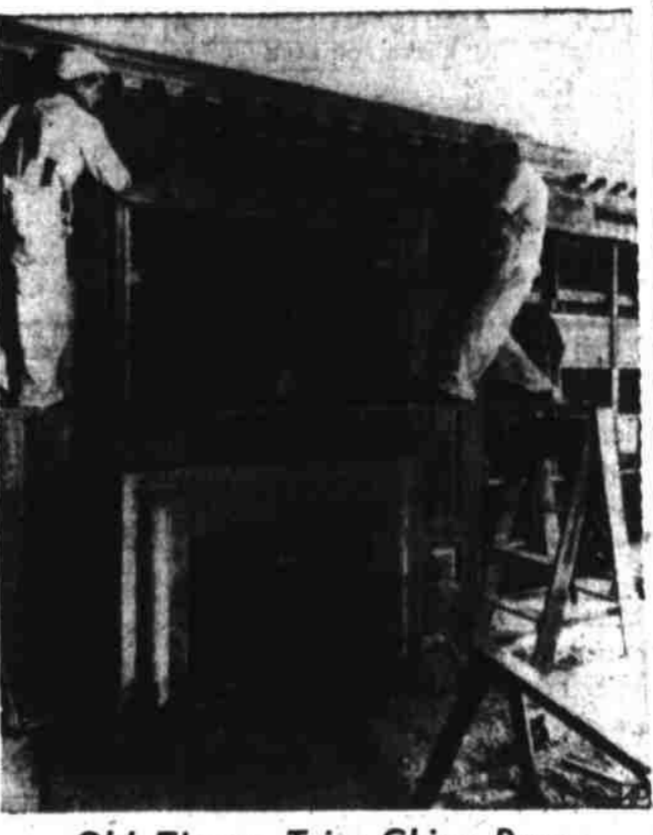
Old Timers Trim China Room Old timbers of the White House, removed during remodeling, are used by workmen for paneling and trimming in the ground floor China Room of the executive mansion. This room was used by past Presidents to display china used on special occasions. The photo made by the Department of the Interior earlier this month, was released by the White House. (AP Wirephoto).
