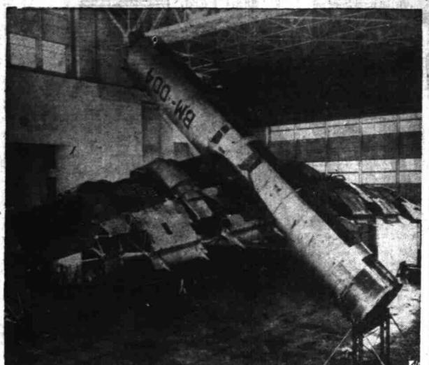
8-36 DELIBERATELY DESTROYED-The Air Materiel Command at Wright-Patterson Field, Dayton, Ohio has begun final destruction tests on the first production model of the B-36, world's largest land-based bomber. Engineers want to determine how much stress weight the wings and fuselage will stand. They will use weights and blocks and tackle to twist the plane into wreckage. The stripped-down craft is pictured being placed on its back for the operation. (AP Wirephoto).
