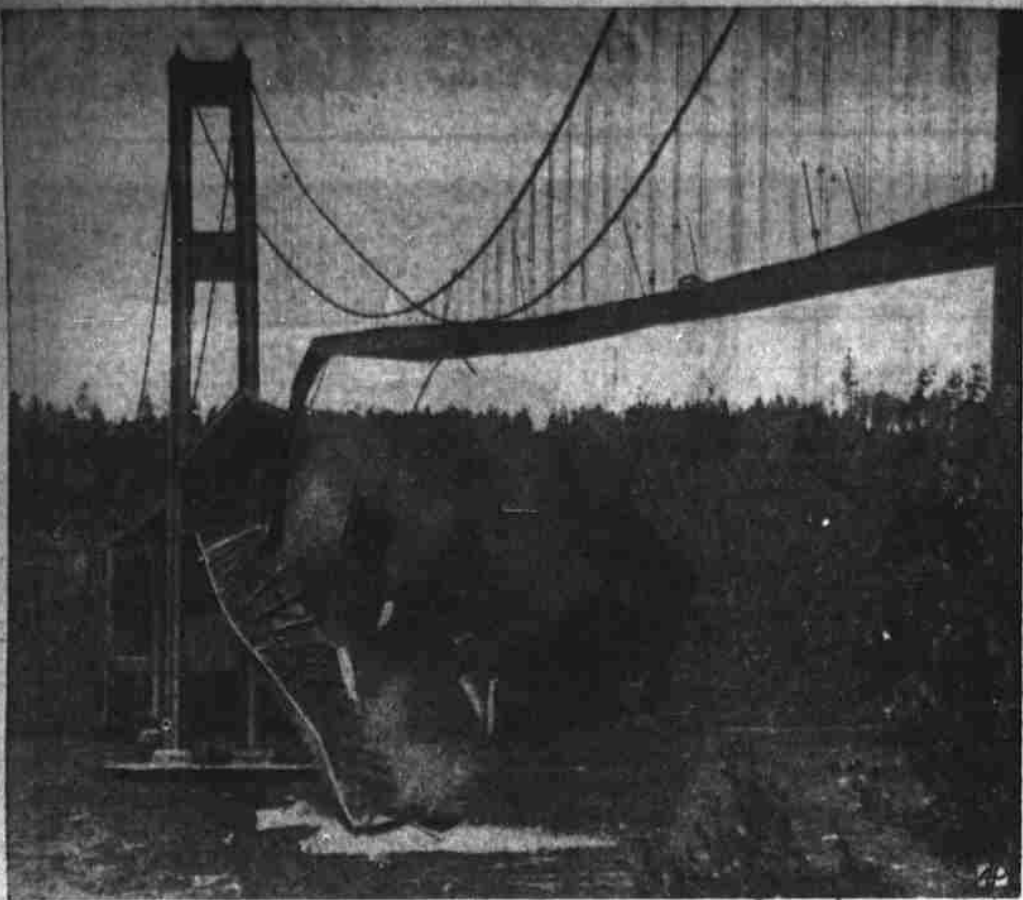
'GALLOPING GERTIE' GOES Wind-blamed crackup of 2,800-foot center span of the new $6,400,000 Narrows bridge at Tacoma, Wash.—third longest single suspension in world—put an end Nov. 7 to the shimmying undulations that gave the bridge its nickname, "Galloping Gertie." Nature's fury in 1940 was also responsible for earthquakes in Turkey (January); Peru (May); Rumania (November).
