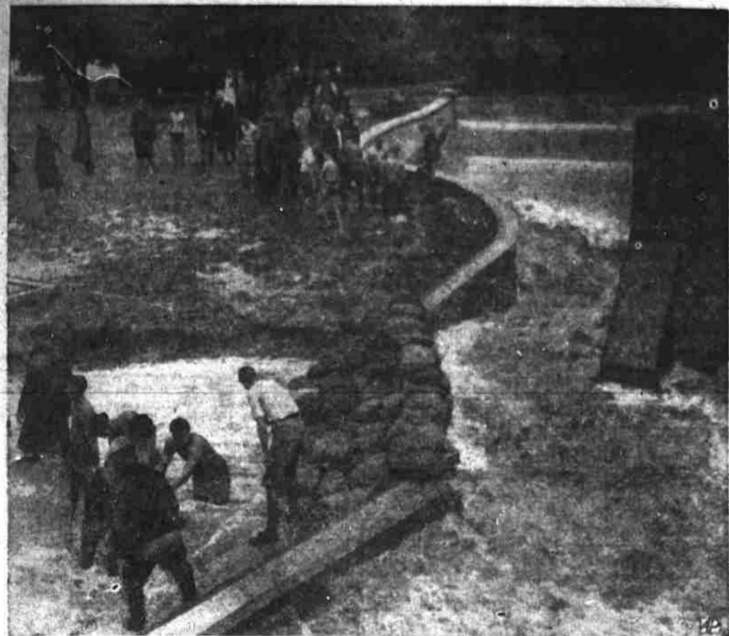
SANDBAGS. AMERICAN STYLE —Knee-deep in water, townsfolk of Clementon, N. J., pile up sandbags to protect the spillway at waterworks lake. This was result of recent Jersey floods.
