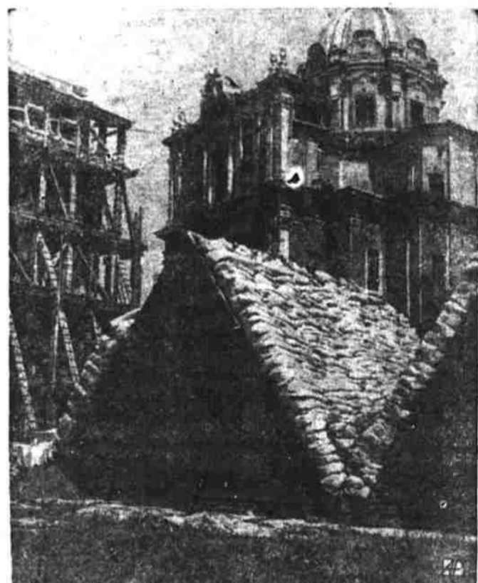
NEW RISK, OLD RUINS —Lest the war machines of modern times add to the ancient ruins with which country abounds, Italy is padding her columns and monuments. This is in the Roman Forum; arch of Septimus Severus is at left.
