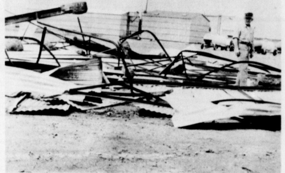
COMPLETE DESTRUCTION is seen as Sandy Sanderson's airplane hanger in Springlake is seen lying in shambles after a freak wind storm Monday night.
