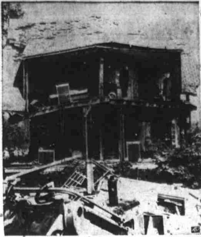
Blast Shatters House
