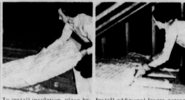
To install insulation, place between joists, press down gently.
