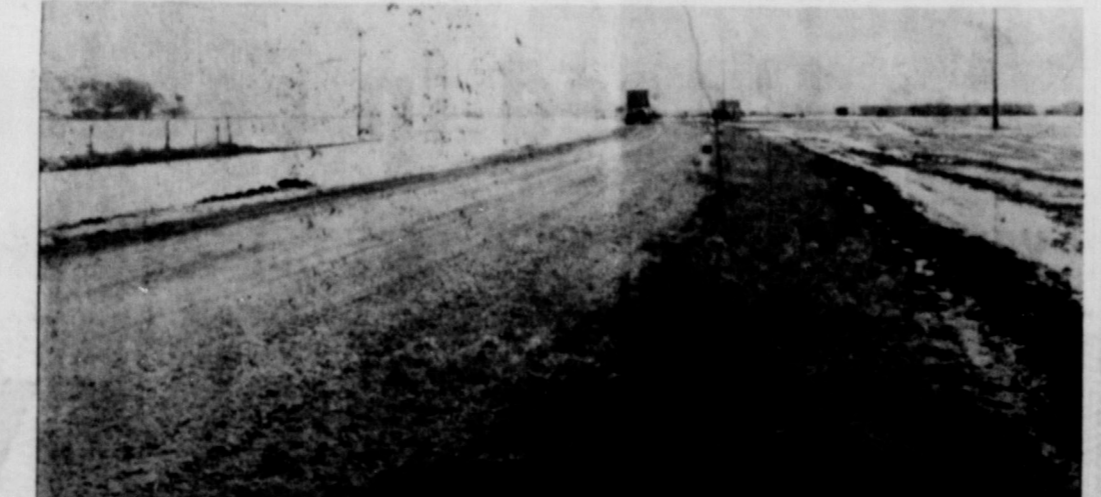
HOW HIGH IS THE WATER MAMA? — Could very easily have been the theme song for many farmers in th area Thursday night after beating rains fell, everflowing fields and damaging crops. Pictured is the north side of Highway 70 showing the F. F. Bozeman farm near the Nickels Gln. Bozeman's crop was damaged, also feed that was stacked in the barn was flooded. In the background is the Ted Robbins residence where water surrounded the house and barns and destroying the fresh cut hay in the fields.
