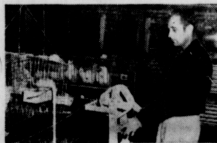
This hand operated rewind reel keeps the fishing string from tangling and keeps it ready to be used again. One length of the string remains in the trough between cleanings.
