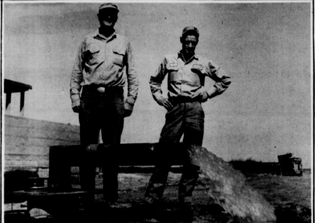
Left to right are Eulis Waggoner of Dimmitt and O. D. Scheller, owner and operator of O. D.'s Pump and Machine Shop of Earth. The water is 350 feet down and being pumped up by this 40 horse power motor.
