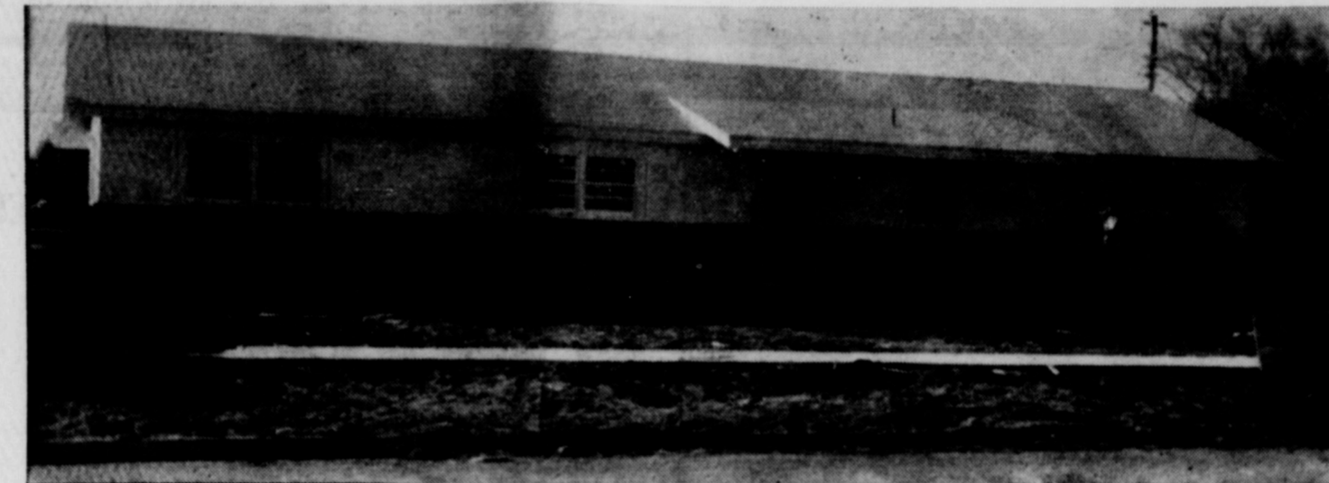
FIRST BRONZE MEDALLION FHA HOME to be built in Earth was built by Trans-Western Developers Inc., Lubbock and Bill Beasley, Earth, local broker. The lovely home of Mr. and Mrs. Charles Crable of 603, second place in Earth has 1,570 square feet of floor space not including the garage. The exterior is of wood
