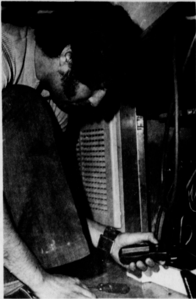
SPC STUDENT WORKS ON UNIT in air conditioning-refrigeration program. Lorenzo Padilla of Earth checks the amp on a soft drink cooler unit constructed by students in the air conditioning-refrigeration mechanics program at SPC. Lorenzo is in his third semester of studies in the program. He and his wife Delores reside in Earth.
