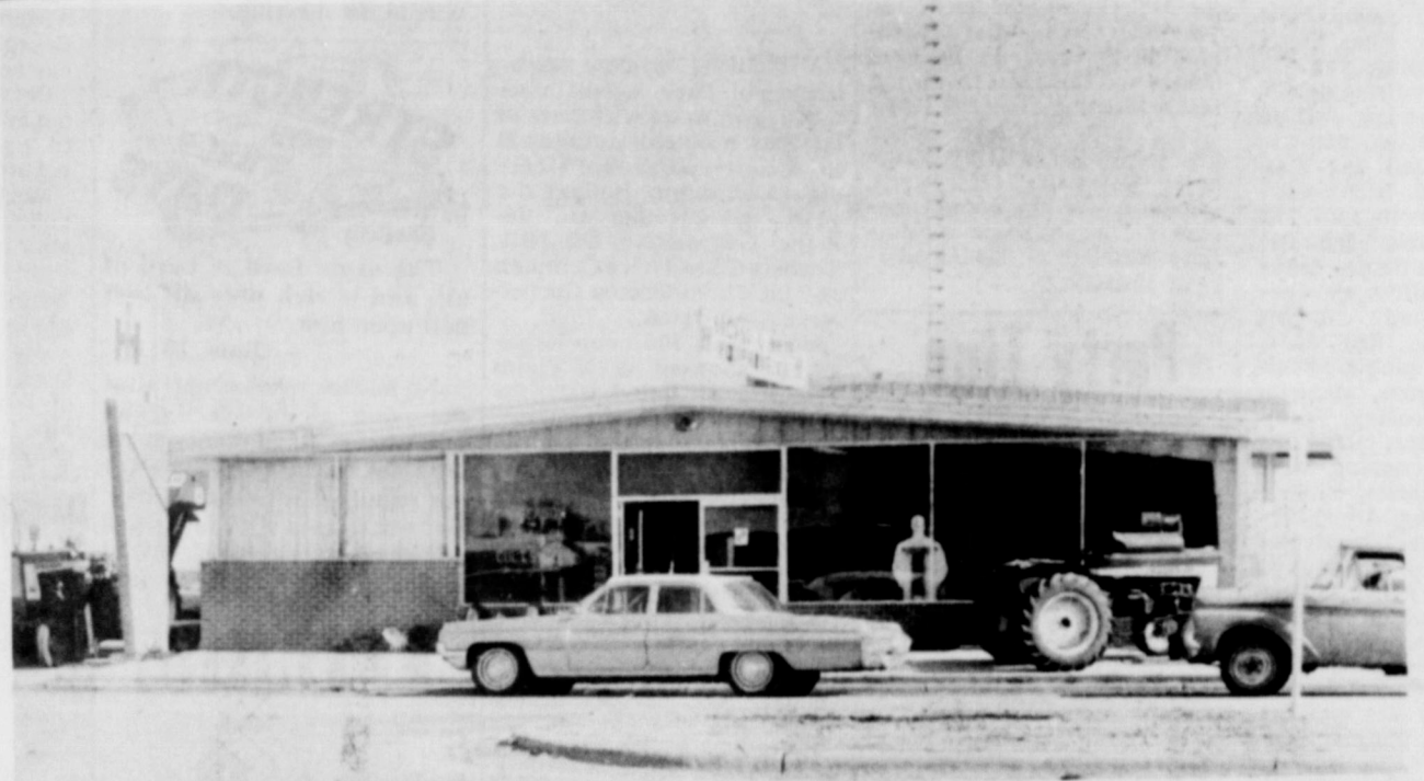
The Brownd-White Equipment Company building, built in 1962. This building is modern and up to date, the crew is anxious and ready to sell and service all International Harvester products.
