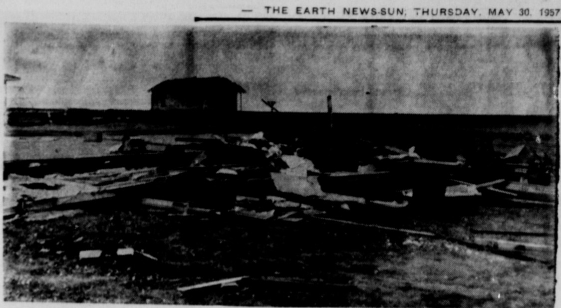
CLASSROOM DEMOLISHED — Pictured are the remains of the old school house that housed the third through the eighth grades where 60 percent of the 50 students enrolled in the two colored schools were having class until 11:50 a.m. when principal B. T. Graves moved the children over to the new brick school building. Desks were placed together in the southwest corner of the building, where students and teachers were placed under desks and tables. All were safe, but the building shook and trembled according to Graves as he watched the destructive mass of wind.
