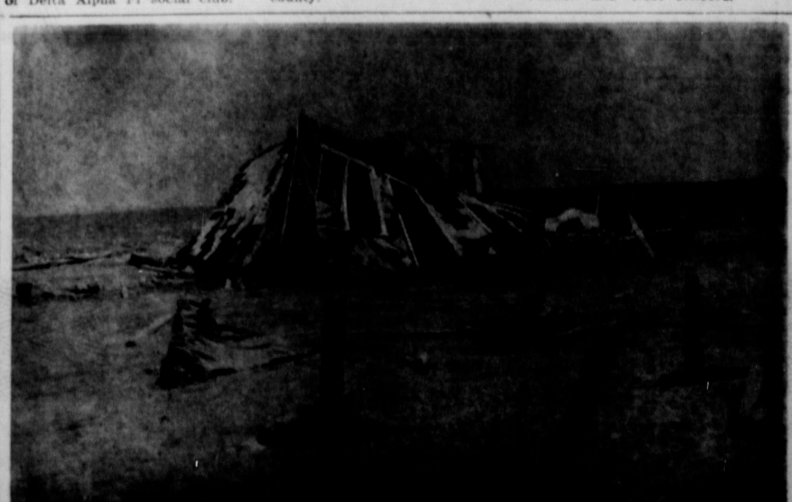
COLLAPSED BY THE STORM — This small residence was only 25 yards from the church where several people sought refuge from the storm. No one was in the building at the time of the storm.
