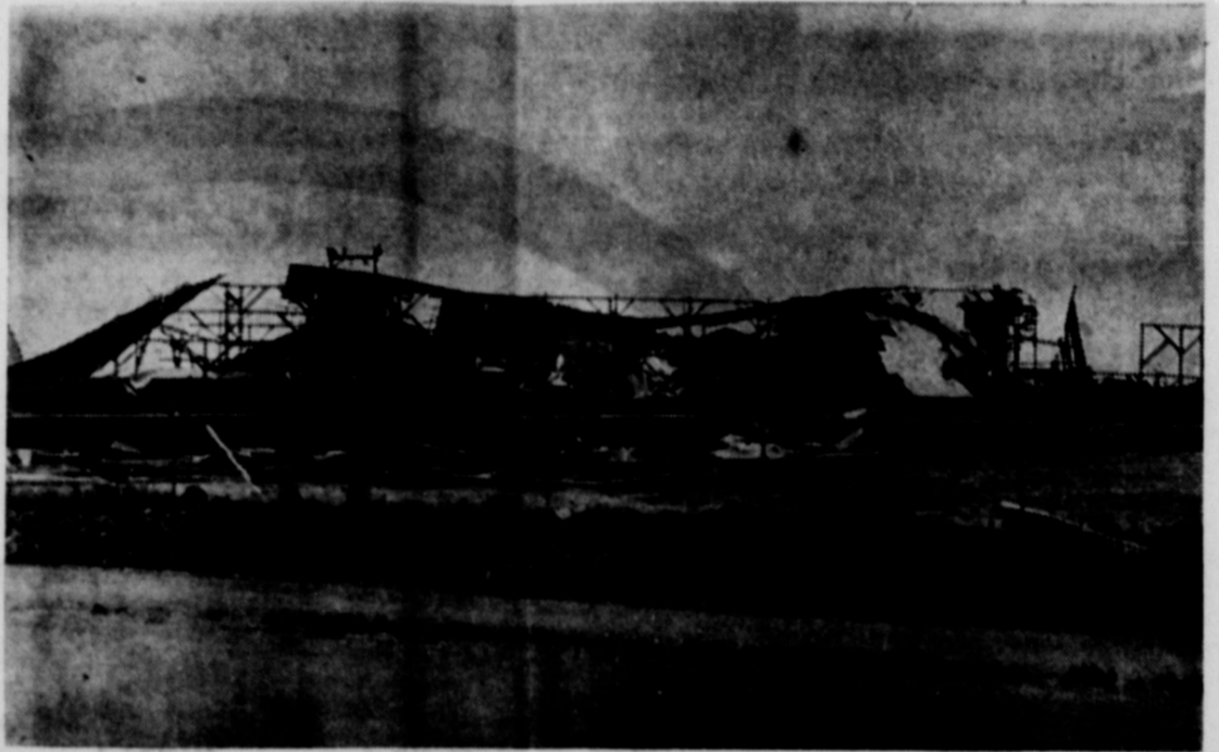
ONE OF THE FIRST BUILDINGS DAMAGED in the storm's path was the Ben Smith Grain Co. elevator. The center section was destroyed. Two employees found safety inside the concrete truck scales.
