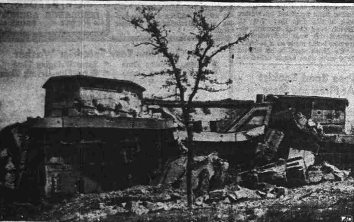
NAZI BUNKER BLASTED —The Zoo Bunker, wartime air raid shelter in Berlin, is blasted by a charge set off by British engineers. Top: The explosion. Bottom: The remains.
