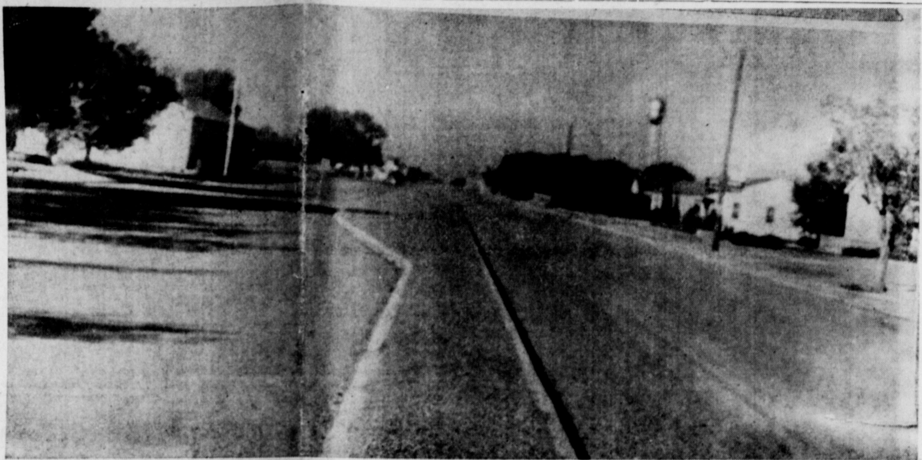
EARTH TAKES ON A NEW LOOK AS THE FOUR LANE STREETS ARE COMPLETED — The widening of Main Street has given Earth the look of metropolitan City. Some of Earth's improvements of the past three years are new business buildings, new sewer system and disposal plant, new housing, new street lights, plus the fact that the town has possibly doubled its population in so short a time.
