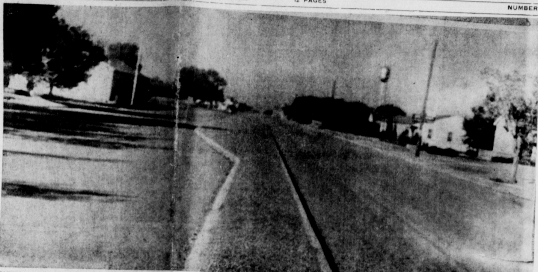
EARTH TAKES ON A NEW LOOK AS THE FOUR LANE STREETS ARE COMPLETED — The widening of Main Street has given Earth the look of metropolitan City. Some of Earth's improvements of the past three years are new business buildings, new sewer system and disposal plant, new housing, new street lights, plus the fact that the town has possibly doubled its population in so short a time.
