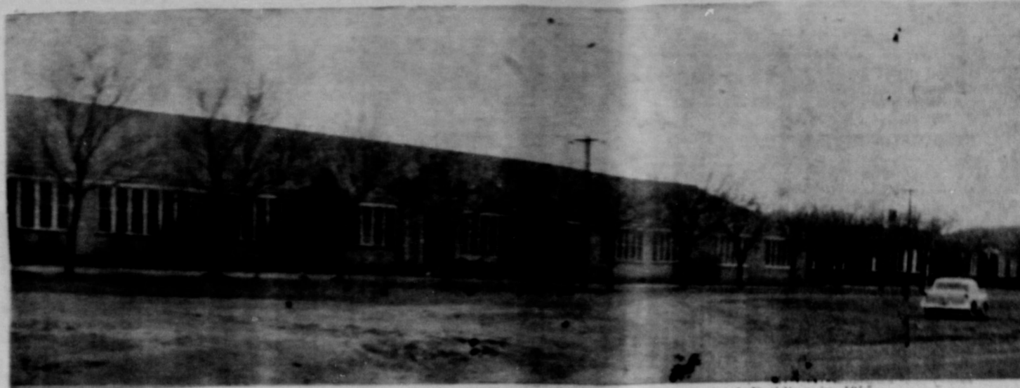
Four new classrooms were added onto the north end of the High School Building in 1955.
