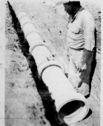
CONCRETE IRRIGATION PIPELINES
