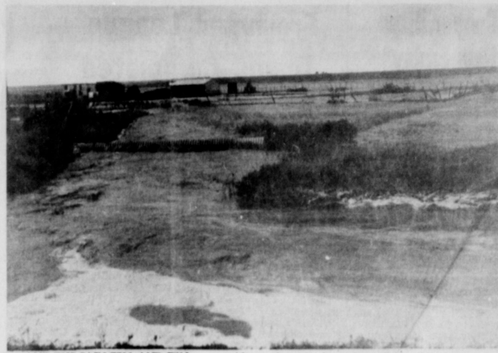
AND THE RAIN FELL AND FELL... as evidence shows in the picture above. The picture was made on the Otis B. King farm east of Springlake, Thursday afternoon, following a heavy rain. Note the culvert in the foreground, where all the dirt has been washed from around it.
