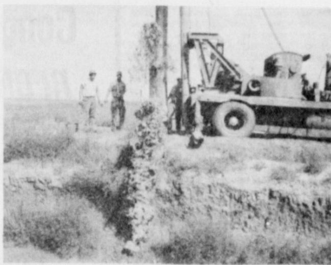
DEVELOPING A NEW HOLE WITH A 30 FOOT, 14 INCH BALER
