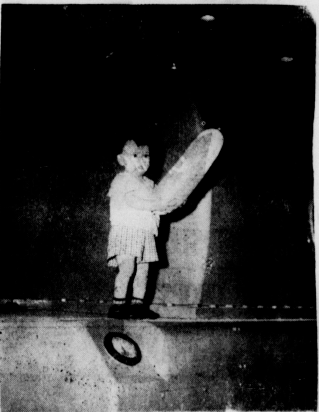
Neal Livingston, son of Mr. and Mrs. Ralph Livingston, and the 112,500 kilowatt turbo-generator recently put into operation at Southwestern Public Service Company's Plant X. Neal holds one of the balloons which were passed out as favors to children of construction men, who were guests at a picnic for construction men and their families at the plant. Neal's father helped assemble and set the giant turbo-generator. With the completion of Plant X, at a cost of $30,000,000, construction men had put in more than 1,500,000 man hours.
