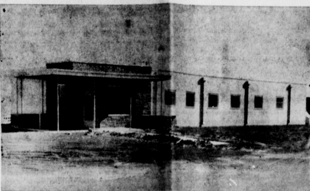
EARTH'S NEW CLINIC — Dr. and Mrs. F. B. Faust are having open house at the New Medical Clinic, located in the East part of Earth, north of the LaCasa Motel, Sunday, January 13 from 2:00 p.m. to 6:00 p.m. The public is invited.
