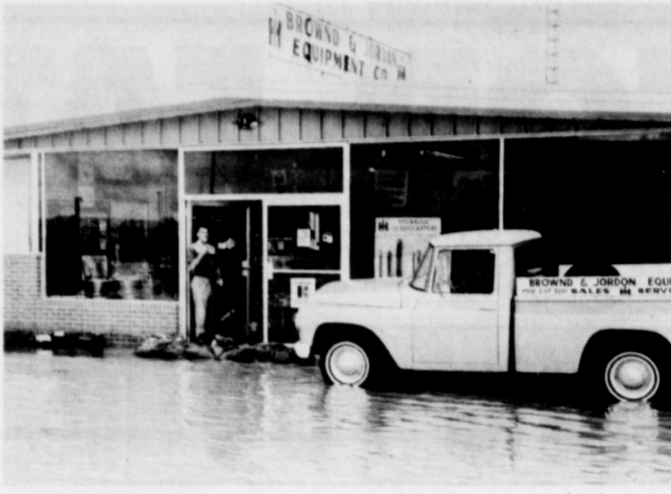
UNESTIMATED DAMAGE was caused by down-pours Wednesday at Brown and Jordan equipment Co., when the building, basement, and warehouse were a deluge of water.
