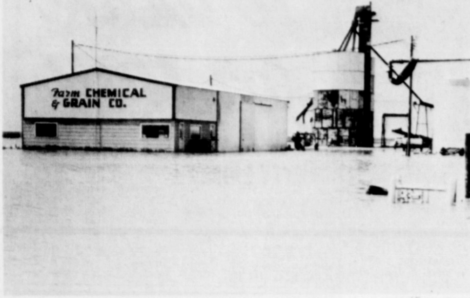
COMPLETELY ISOLATED, Farm Chemical Grain Co. stands alone on its' own little island as a result of rains last week which brought approximately six to eight inches to the area. Damage to fertilizer, seed, and other merchandise has not been estimated, but is expected to run high.
