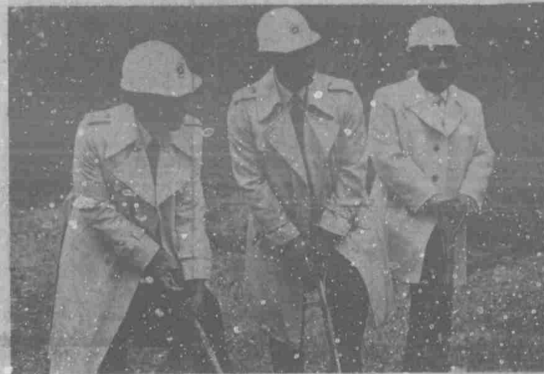
NAPFE BREAKS GROUND (Chattanooga, TN) -- Robert Williams, Robert L. White and Alonzo Adams of the National Alliance of Postal and Federal Employees (NAPFE) break ground for a $5.2 million elderly housing complex in Hamilton County, Tennessee. The Chattanooga NAPFE Elderly Housing Complex which is financed through a U. S. Department of Housing and Urban Development (HUD) Section 202 low interest loan is designed as a nine-story 124 unit apartment building with an 80-seat dining room, lounge and game area. The building will be ready for occupancy in early 1983. (Photo by Jacquelyn C. Moore)
