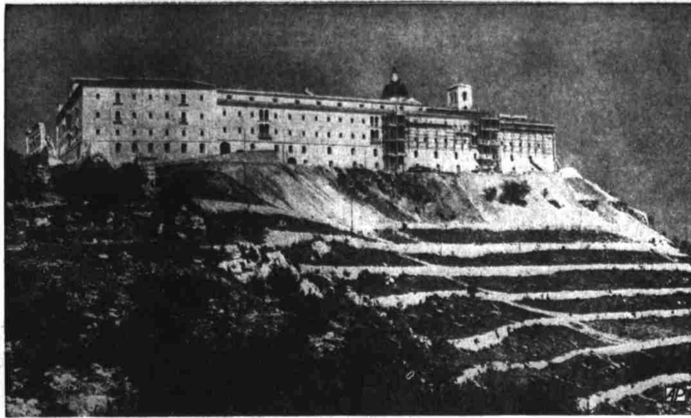
MONTE CASSINO RISES AGAIN —The ancient historic Benedictine Abbey of Monte Cassino, familiar to thousands who fought their way through Italy in World War II, presents this rebuilt face following extensive post-war repairs.
