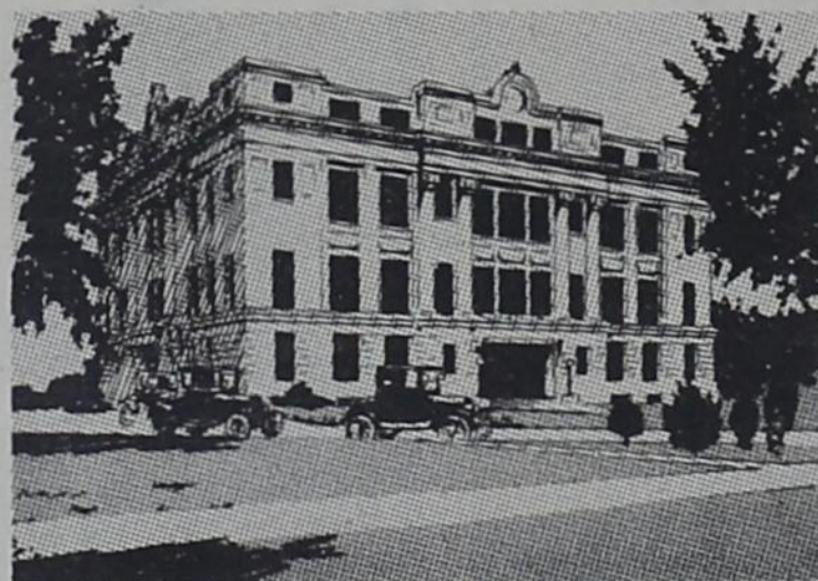
The Old Lubbock County Courthouse, Built in 1916.
