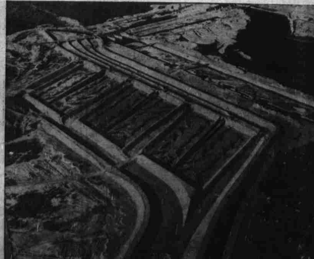
LIKE A CHILD'S SEASHORE PATTERN in the wide, desolating works of the All-American canal stretch in symmetrical design on the California side of the Colorado river at Imperial dam. Here, all-laden water will be clarified before it is directed to the canal (in foreground) on its 90-mile journey to the irrigated Imperial and Coachella valleys.
