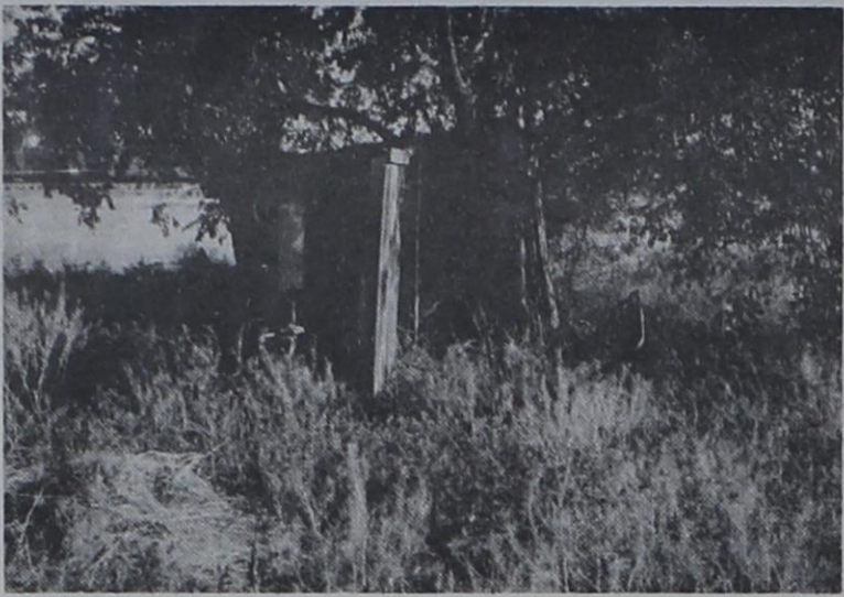
FIRE HAZARD IN COMMUNITY —An old outdoor privy and a shack, surrounded by dried weeds, is one of many fire hazards in East Lubbock, as can be seen in this photograph. This structure is found at 2403 Globe Avenue. Although the lot does not belong to Urban Renewal, the owner should be made to cut the weeds (according to a City Ordinance) and remove the unsanitary facilities. (Staff Photo)
