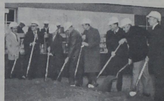
NOV. 29 GROUNDBREAKING . . . AND CONSTRUCTION MOVES AHEAD
