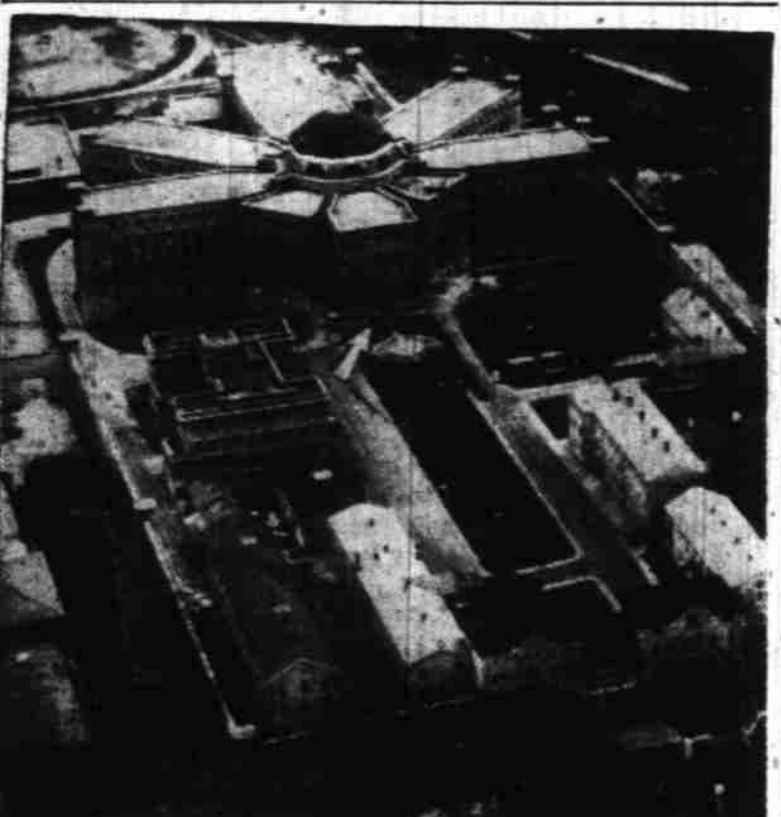
WHERE PRISONERS RIOTED—This is an aerial view of the U.S. Disciplinary Barracks at Ft. Leavenworth, Kas., where about 800 prisoners rioted. One inmate died in the disturbances. The main entrance through the wall is in the center foreground. Note main entrance door to building entering cell block area (arrow). (AP Wirephoto).
