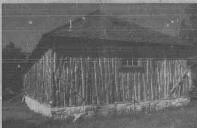
Shown here is the Palisado Building that the Texas Tech Upward Bound students helped document at Fort Clark in Brackettville. The building was built by 25th Infantry Buffalo Soldiers in 1869-70.
