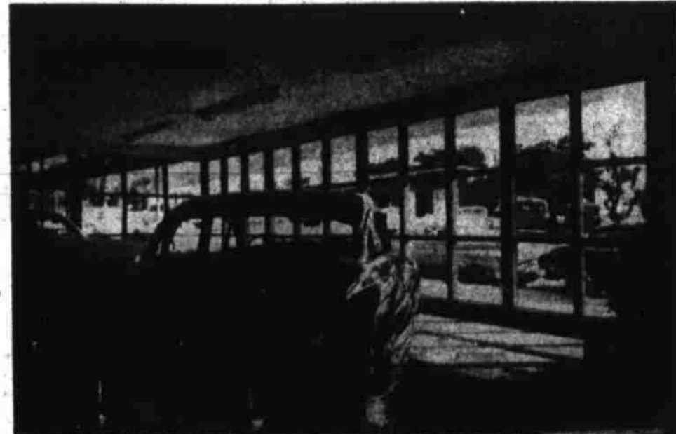
We Are proud to have installed the plumbing, Plumbing Fixtures and the hydraulic lifts in this new and modern building in Big Spring.
